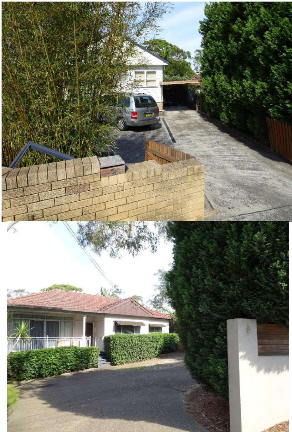
Figure 3a: Photograph of 2-4 Anzac Avenue in Engadine
